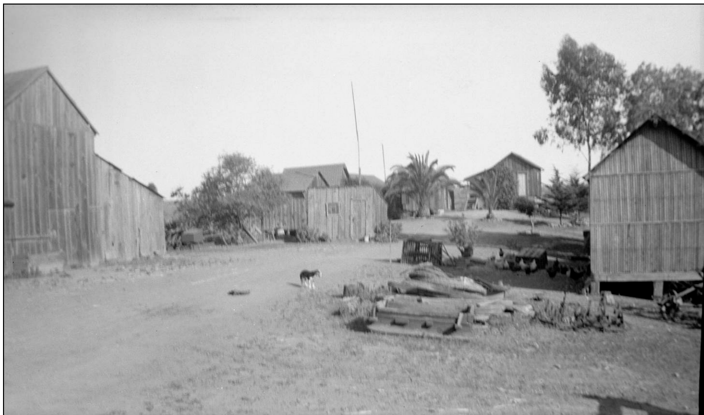
Figure 7. Ranch Yard and Buildings with Homestead Shanty (center), view south, 1936
